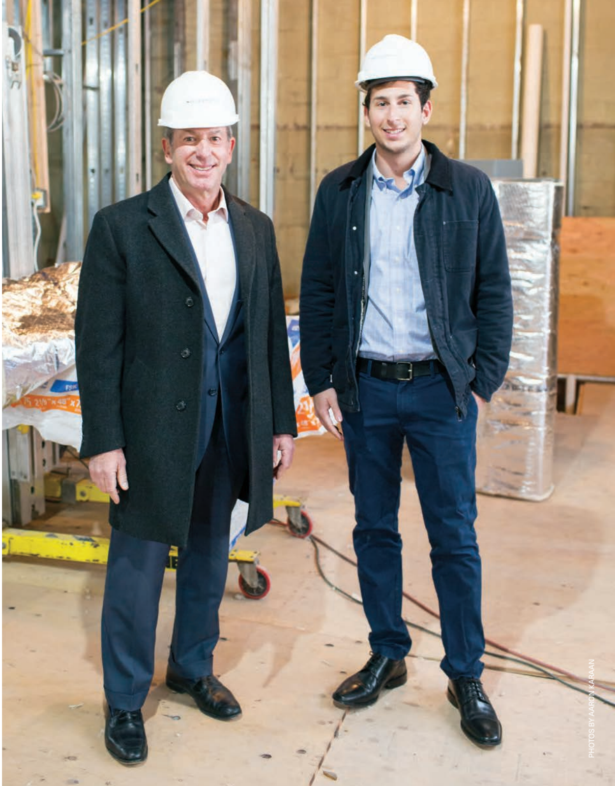
Paul Silverman '78 (left) and Justin Axelrod '20 were all over Jersey City during Axelrod's four-day externship. Here, they visit the construction site of a future SILVERMAN property.
